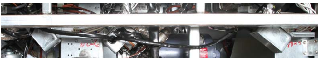
Figure 24: Outlet boxes shown in place on a LOV fryer with power and heater tapes connected. OCF fryers don't use the center junction box.
