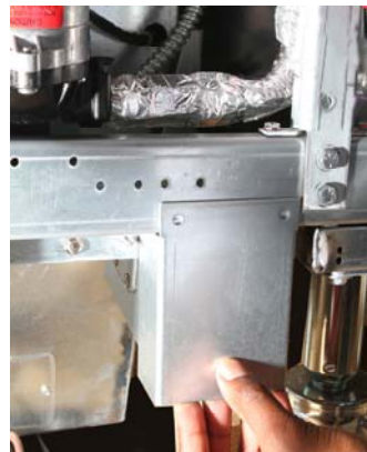
Figure 18: Position the thermostat protective cover over the thermostat and mount with drill-point screws.
