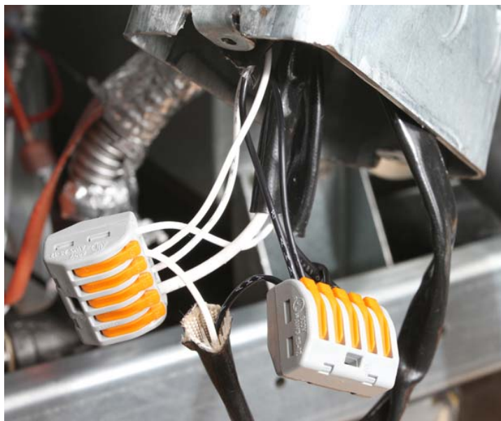
Figure 23: Wago connectors shown in junction box.
