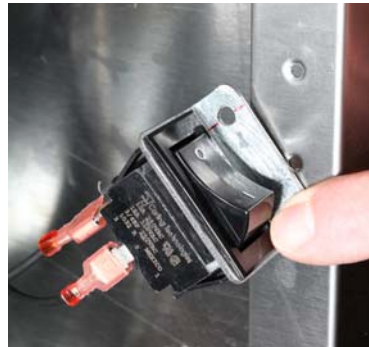
Figure 14: Switch being positioned on JIB cabinet right interior (front view).
